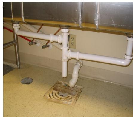
Section 5-402.11 of the Missouri Food Code Prohibits a direct connection between the sewage system and a drain originating from equipment in which food, portable equipment, or utensils are placed.
