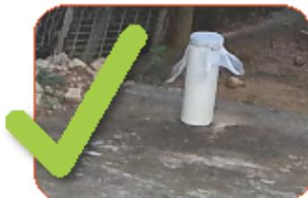
Septic tank ventilation pipe with screen mesh
