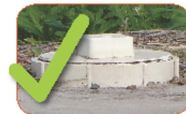
Septic tank sealed with PVC cap
